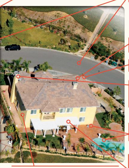
**Walls:** Wood products, such as boards, panels, or shingles are common siding materials. However, they are combustible and not good choices for fire-prone areas.
